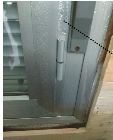
humidity in aluminium carpentry
